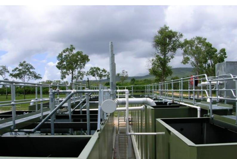
Hydroflux Epco RoadTrain® packaged sewage treatment system delivering high quality effluent for environmental protection
