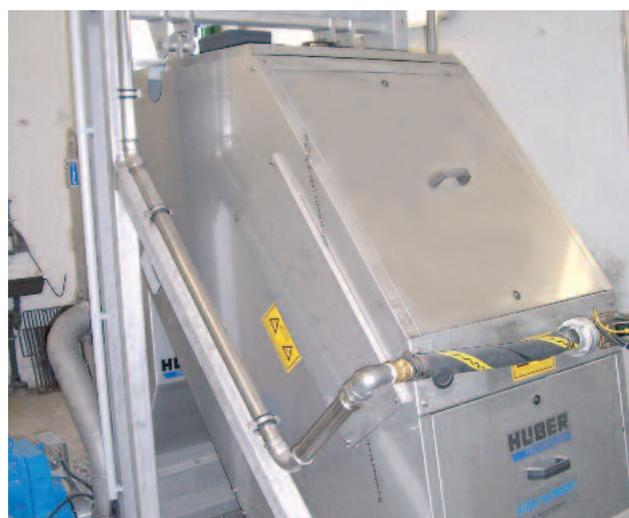
Fully enclosed, odour-free STEP SCREEN® Flexible SSF
