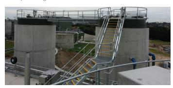
The gas covers were provided with the necessary ancillaries, such as the ballasts, sight port assemblies, sample hatch covers, pressure/vacuum relief valves and emergency relief valves.
