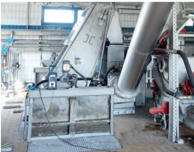
The HUBER Multi-Rake Bar Screen RakeMax® CF is an universally applicable screen for both new and existing structures.
