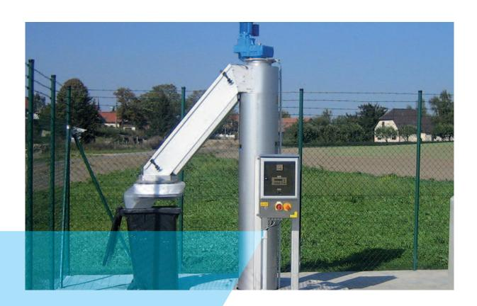
Automatically cleaned fine screen with vertical lifting, dewatering and compaction of screenings
