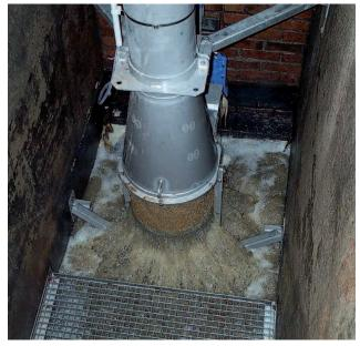
ROTAMAT® Pumping Stations Screen RoK 4 in operation
