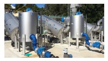
The technology installed is the HUBER Rotary Screw Thickener. This process uses an internal screw housed within a wedgewire drum.
