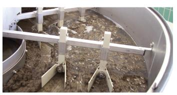
The thickened sludge is stored in a fully mixed short span retention tank and then is dosed with a polymer and is dewatered in a HUBER QPRESS.
