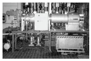
The total mixed sludge is screened immediately before the heat exchangers. The fibrous material and hair are separated from the sludge flow and compacted. 60 m<sup>3</sup>/ hour of mixed sludge are fed into the STRAINPRESS® by gravity or vacuum forced through the machine by pumps behind the coarse material separators. The inlet concentration of the primary sludge is between 2 and 3% DR.
