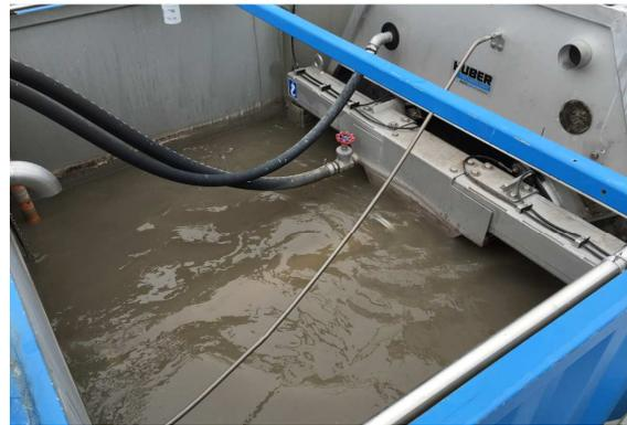
**Fig. 8: Flow to the *HUBER Drum Screen LIQUID* with maximum upstream water level [8]**
